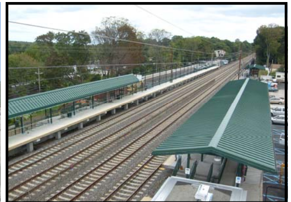
SEPTA Wayne Station; Wayne, PA Architect: Systra Consulting, Inc.
