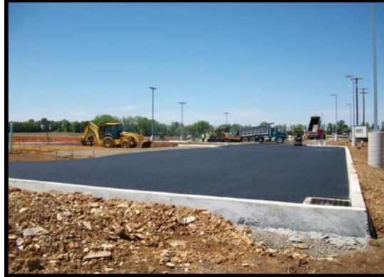
Trexlertown Development ; Lehigh County, PA Engineer: Landcore Engineering Consultants
